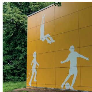
Lübeck – site of the Falkenfeld elementary school and gymnasium. To make its purpose apparent from the outside, images of athletes were applied to the facade. The dynamic motifs were cut out from the film with a cutting plotter.
